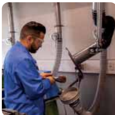
Extraction arm at the grinding workplace
