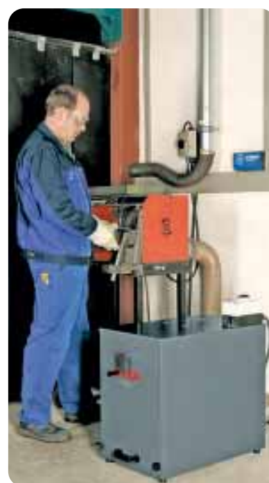
Mini dust collector TK connected to a deburring machine
