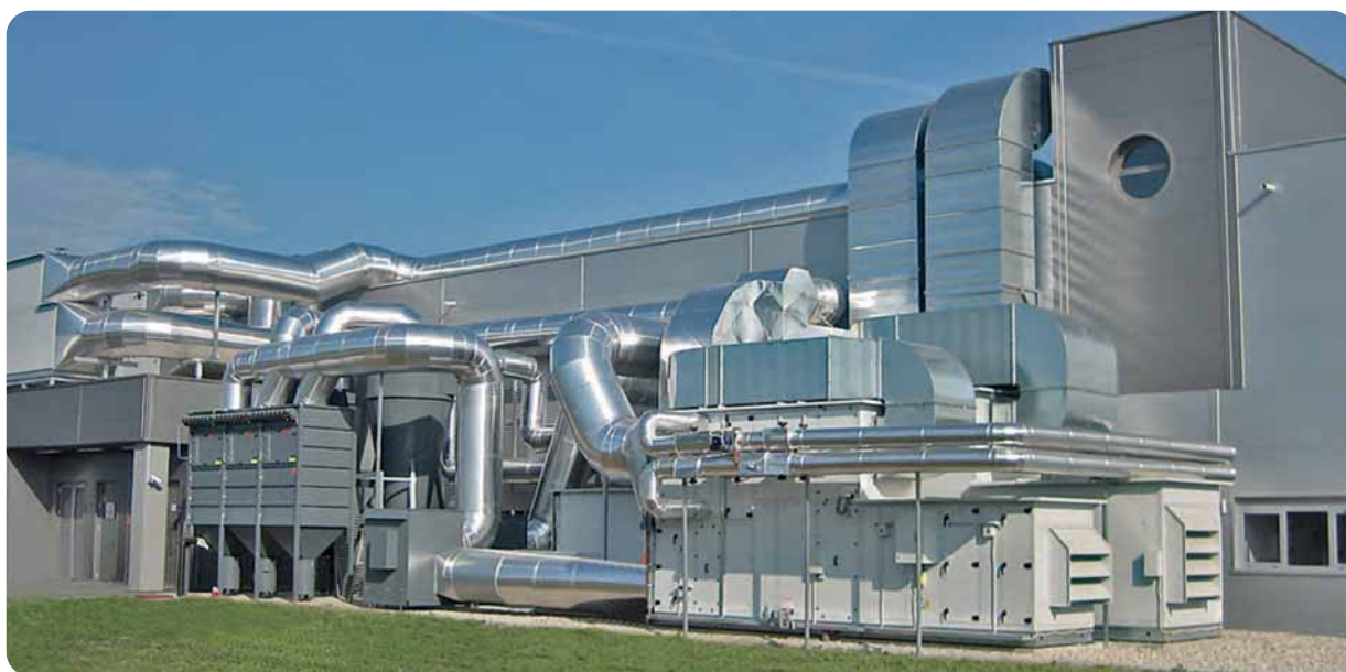
Individual plant concept with DUSTMAC filter units in the shoe industry
