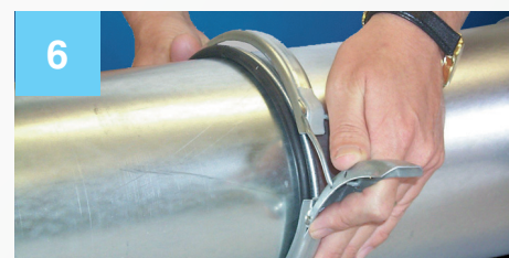
6 Snap QF clip over the O-ring and one end of the slip duct
