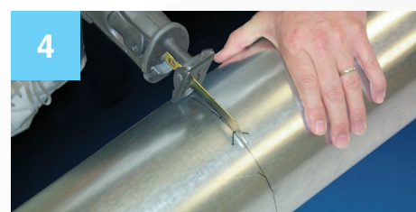
4 Cut the duct.
