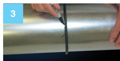
3 Use O-ring provided and mark for cut.
